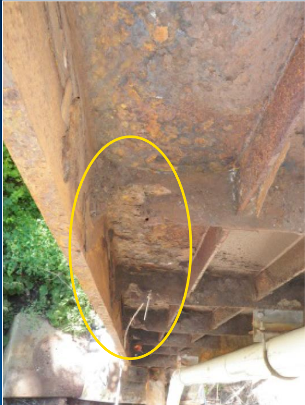
Source: 2013 inspection report
