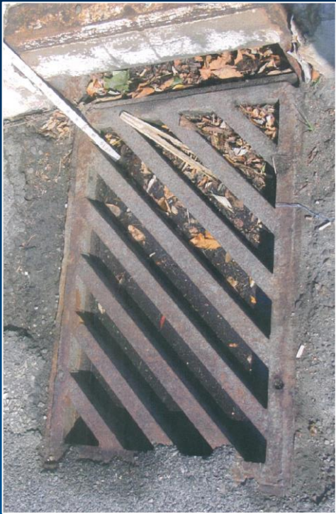
Source: 2005 inspection report
