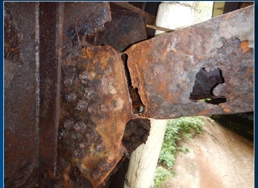
Source: 2021 inspection report
