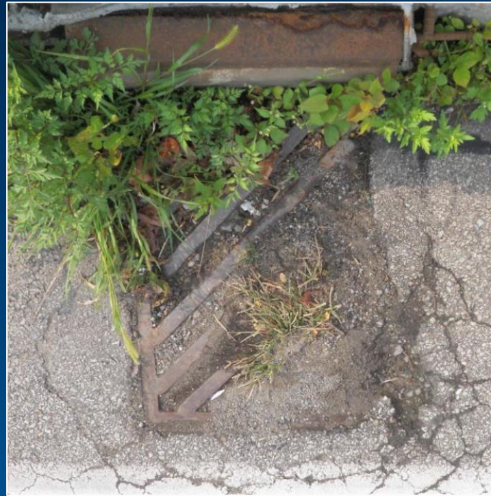
Source: 2017 inspection report
