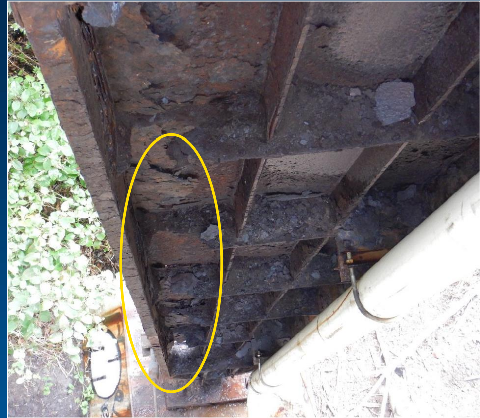
Source: 2021 inspection report
