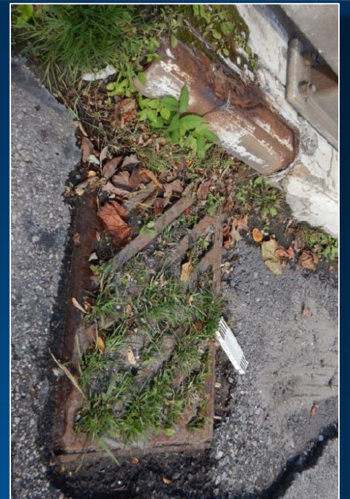
Source: 2021 inspection report
