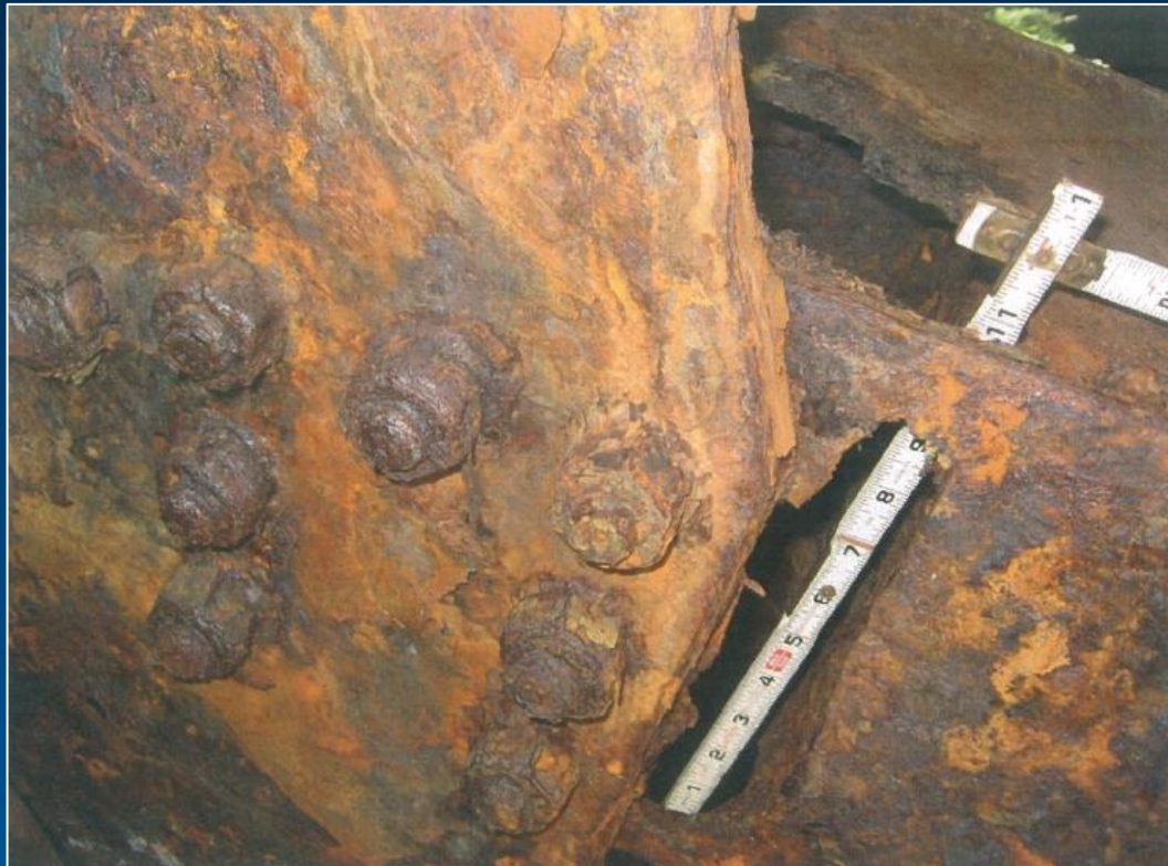
Source: 2005 inspection report
