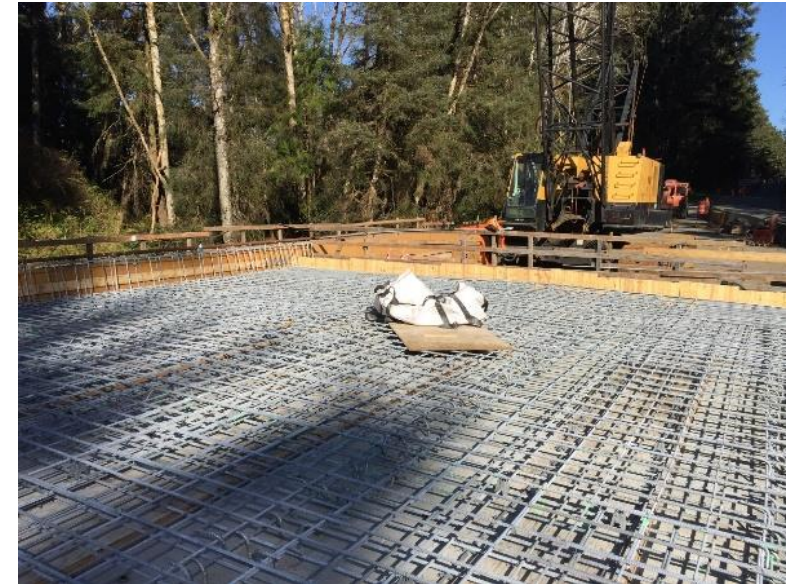
Galvanized rebar in Washington
