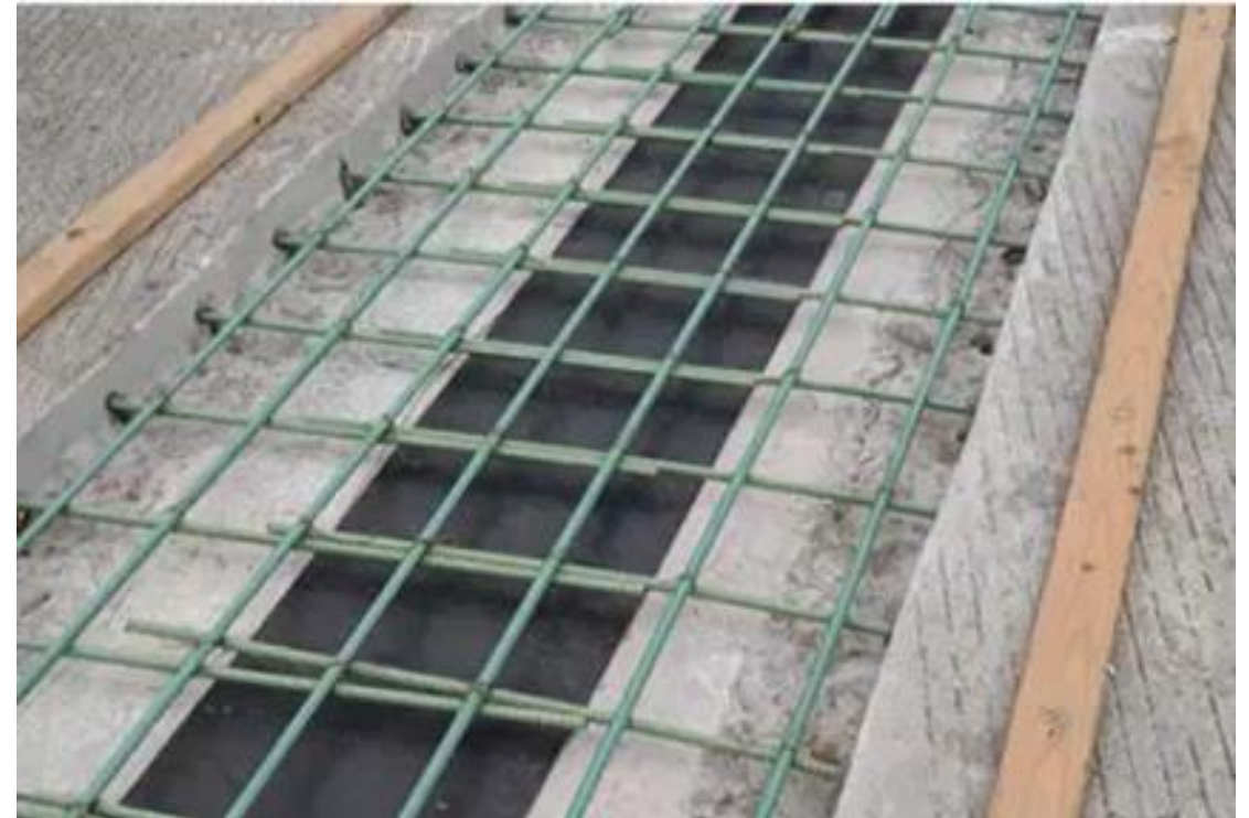
UHPC link slab from New York
