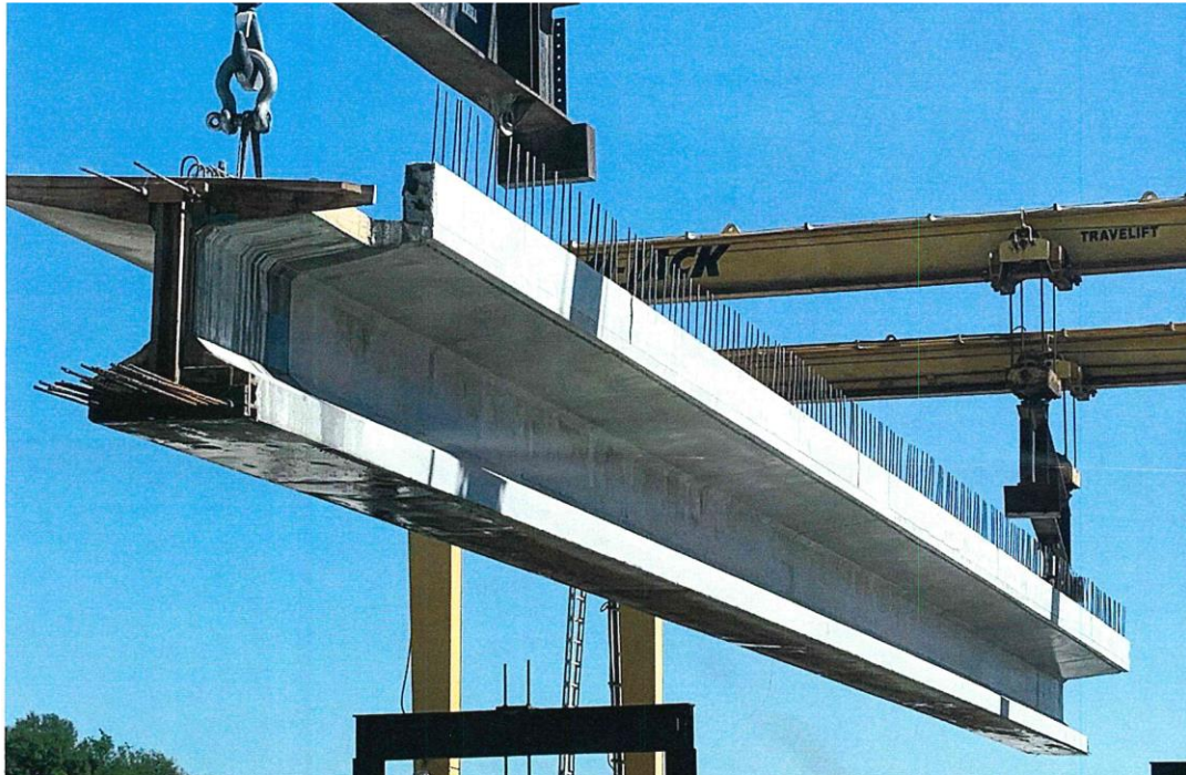
Precast deck overhang in Texas
