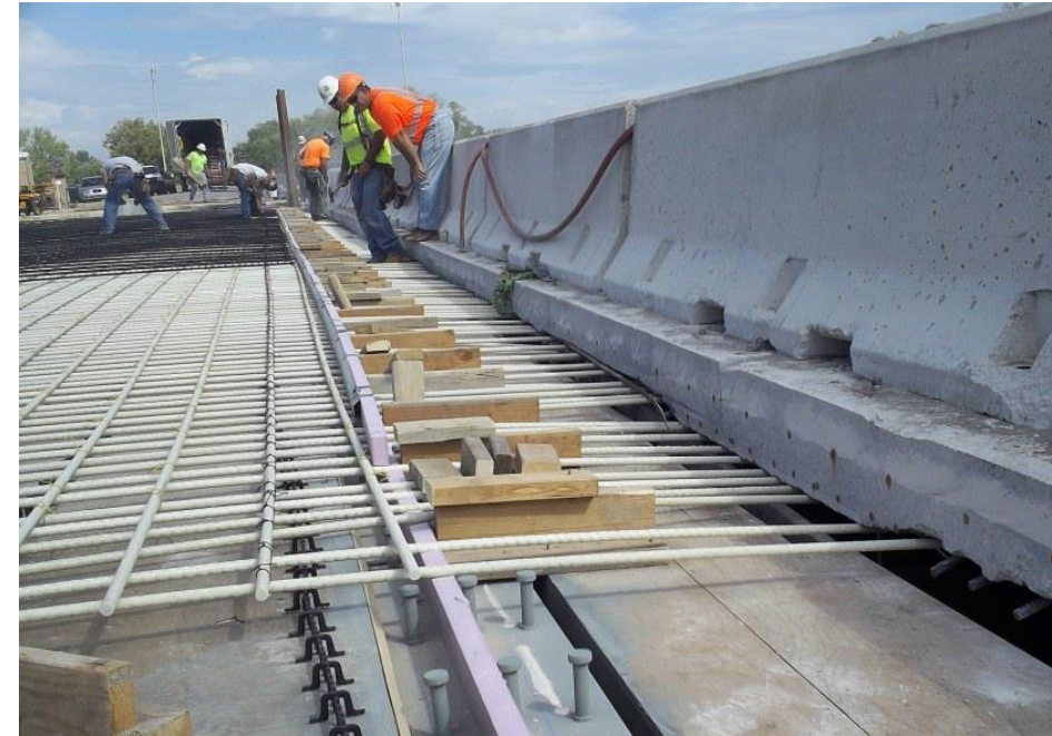
Glass FRP bars in a deck from Kansas
