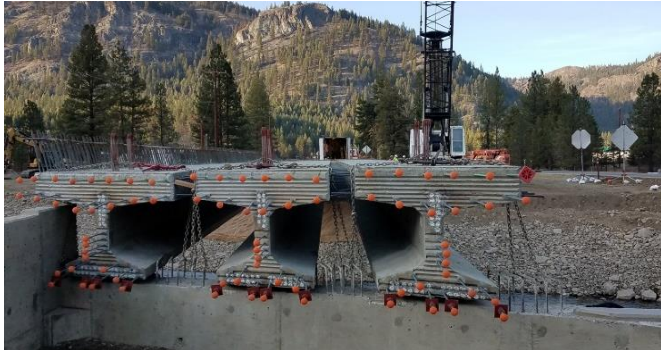
Decked girders in Washington
