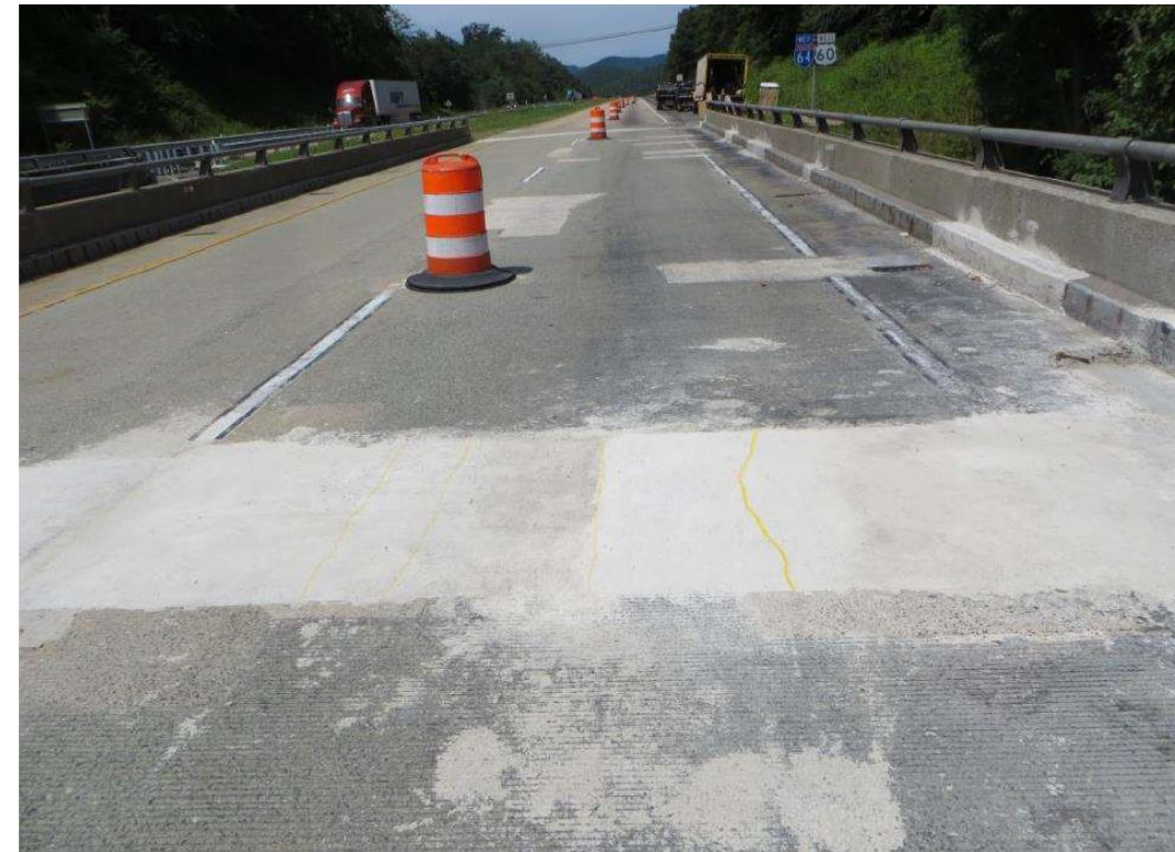
Fiber reinforced concrete link slab from Virginia
