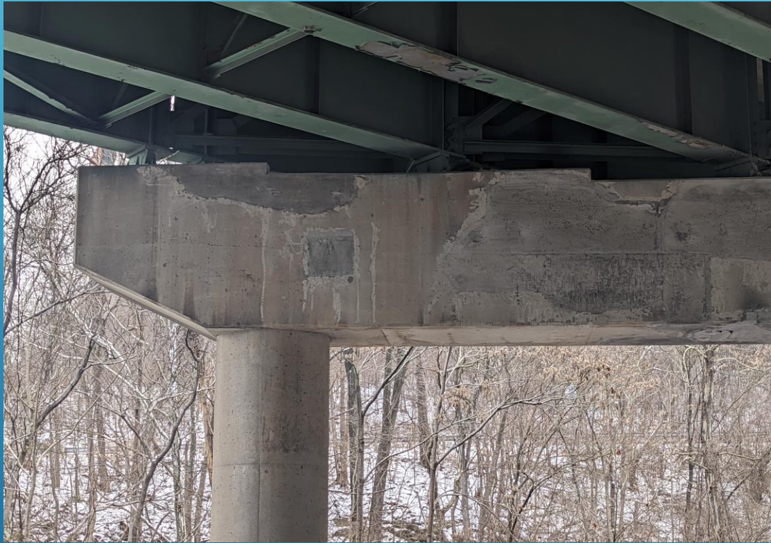
Uncoated Repair Surface
