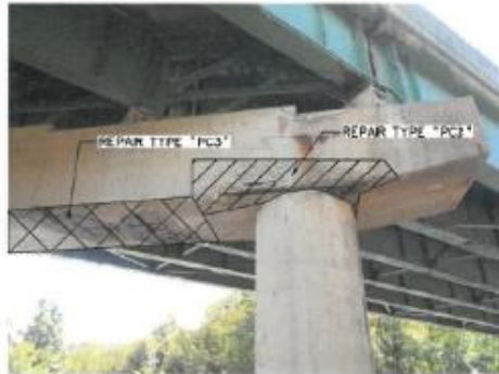
NB PIER 3, NORTH FACE
