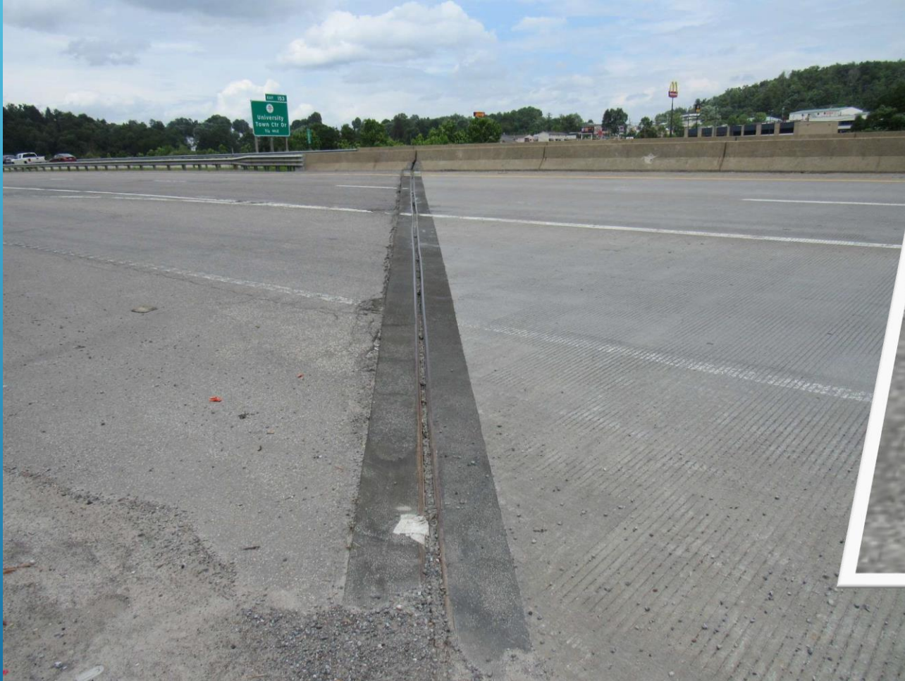
Typical Strip Seal Expansion Joint in this bridge.
