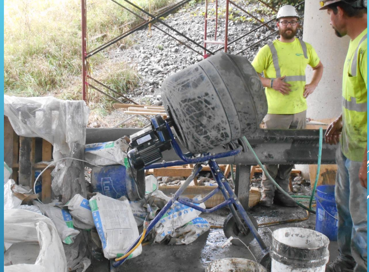
Mixing Rapid Set Cementitious Patching Material (on Site)
