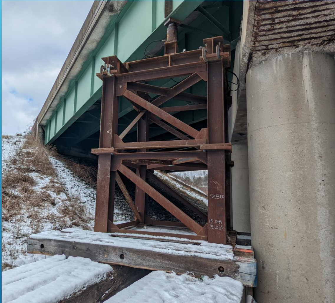
Jacking Tower (North Side of Pier)
