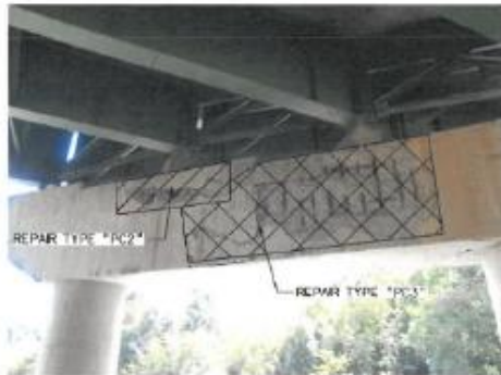
NB PIER 3, NORTH FACE
