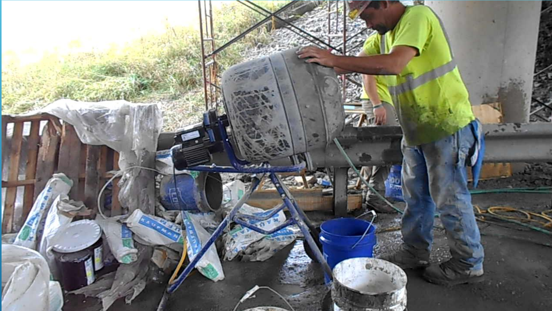
Site Mixing of Rapid Set Cementitious Patching Material
