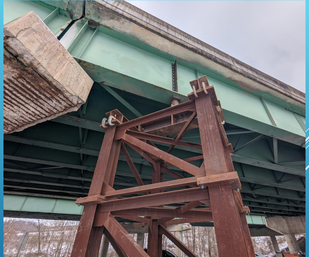
Jacking Tower (South Side of Pier)
