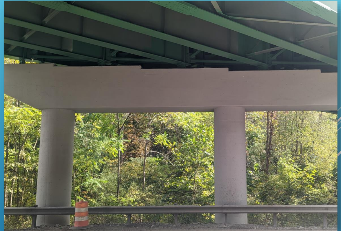
Coated Repair Surface
