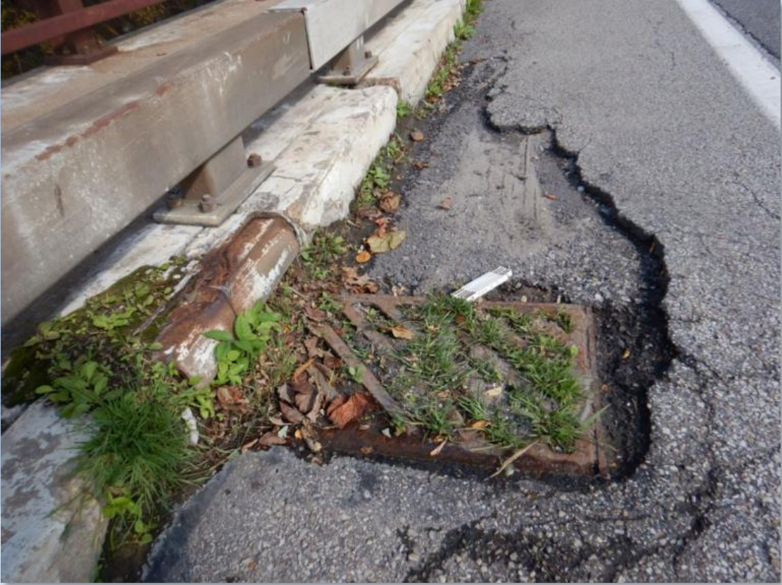
Old Fern Hollow Bridge (September 2021)
