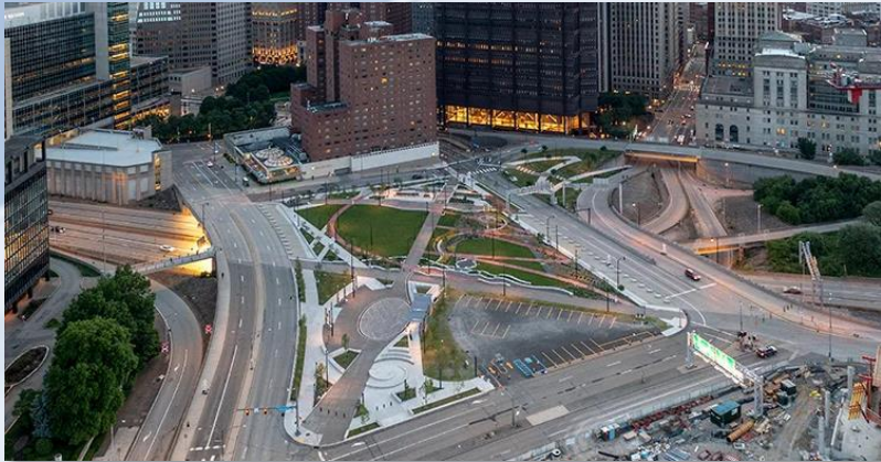
Frankie Pace Park- Cap over a 1960's era "urban renewal" highway
