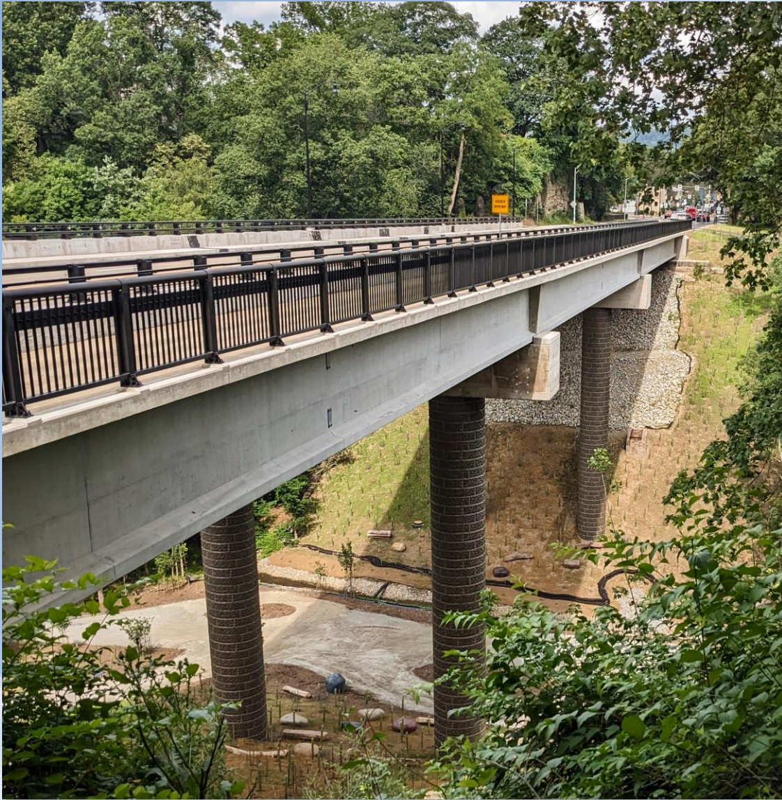
The new Fern Hollow Bridge (2023)
