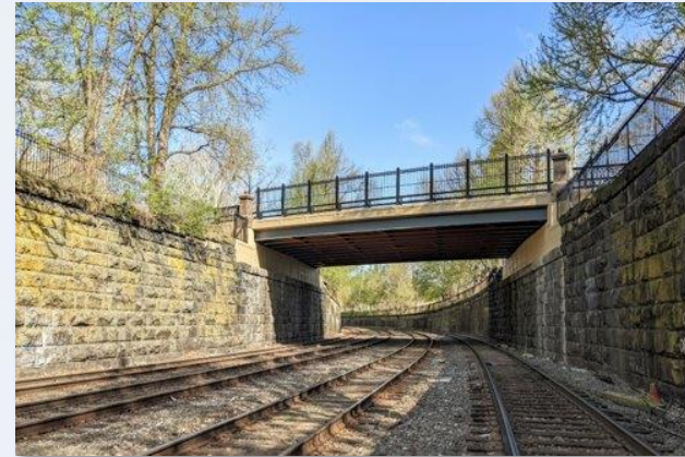
West Ohio St- Replaced 117 year old pony truss
