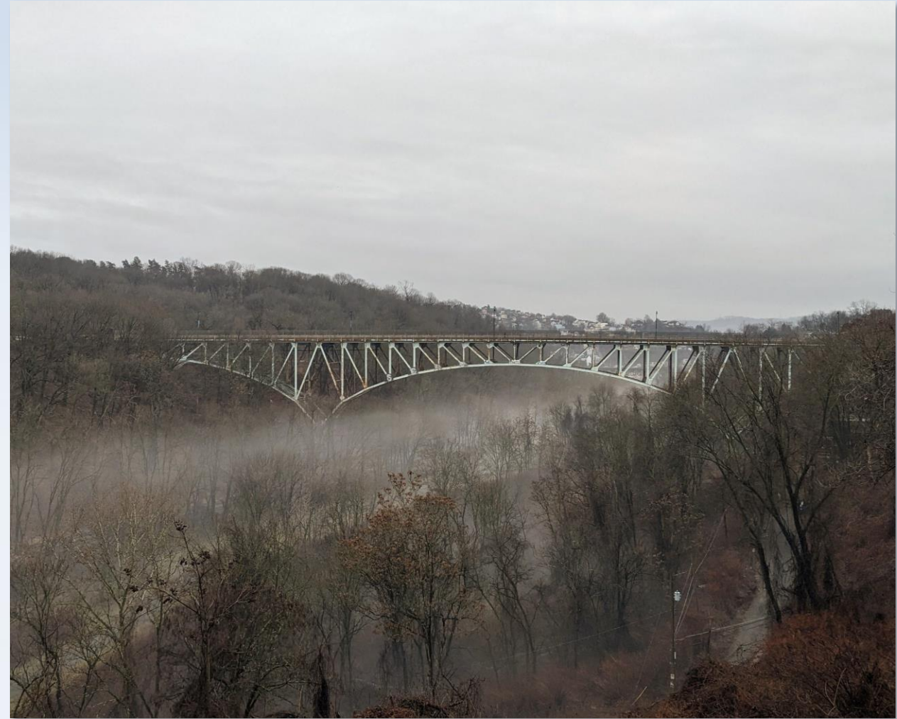
Charles Anderson Bridge, built 1939
