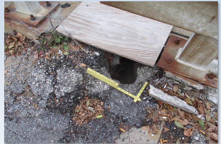
Elizabeth St Bridge, before...
