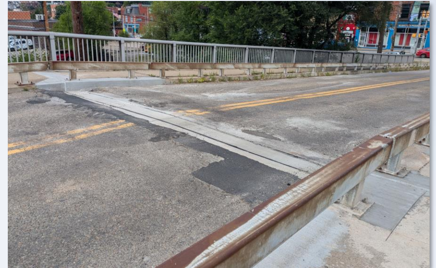
Elizabeth St Bridge, after!
