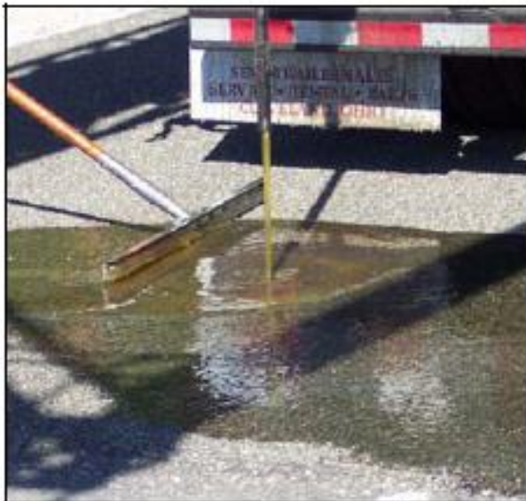
Crew uses squeegee and roller to distribute product across deck.
