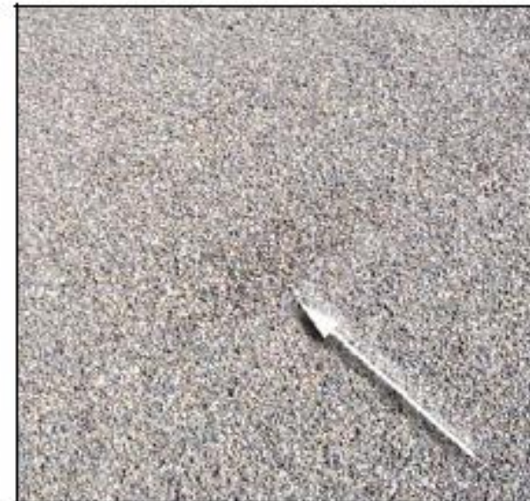
Material is disbursed by hand to areas where epoxy comes through.
