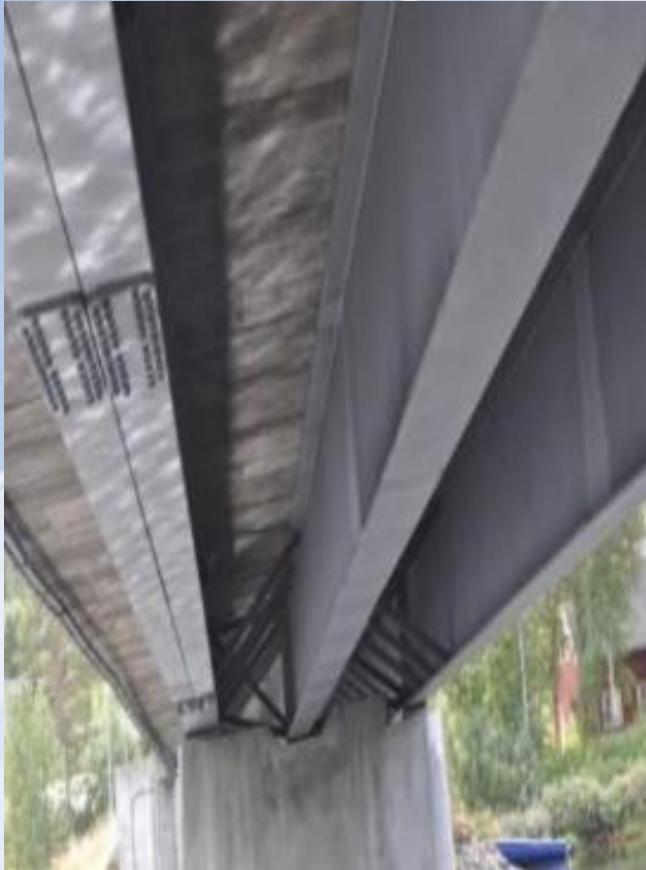
The 'Seims Bridge' in Norway after 30 years of service. Both the inner and outer faces are in perfect condition.
