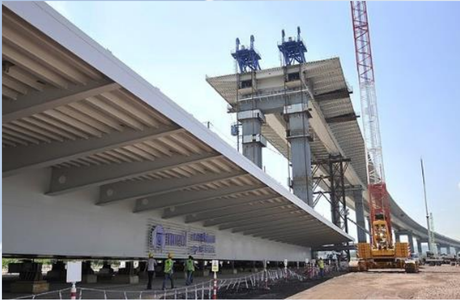
The 'Ozmangazi Bridge' under construction
