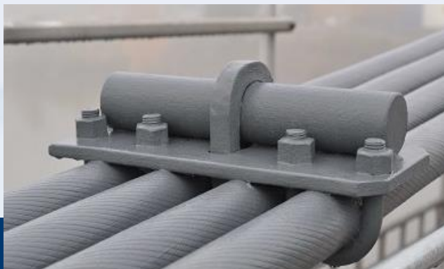
Bridge cables on Kalvoya Bridge, Norway
