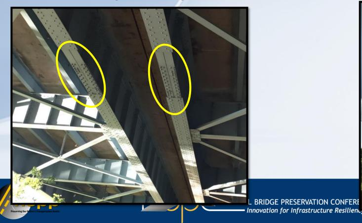
Pin and hanger - 4 locations per girder (~0.5% of girder length)
