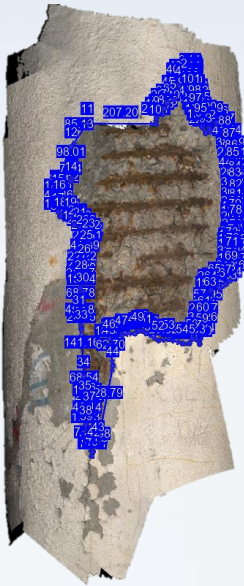
Concrete spalling
