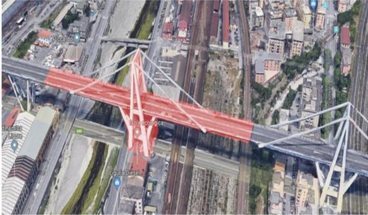
Pillar 9 that collapsed
