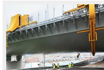
— Pic #8: Cameras on the Retractable Beam of the RobotInspection (from Camozzi)
