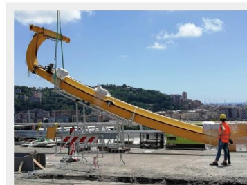
— Pic #9: Size of the Transversal Beams of the RobotInspection (from Building CuE)
